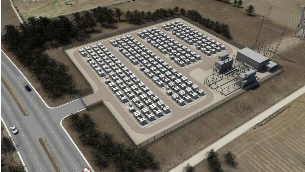
Tesla Grid Storage Facility (Southern California)
