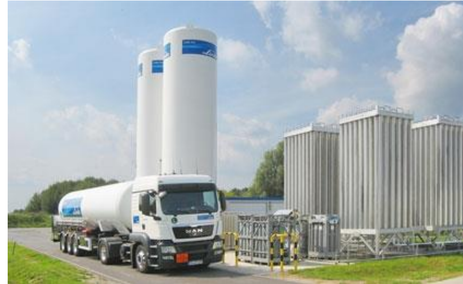
Liquid hydrogen trailer:
