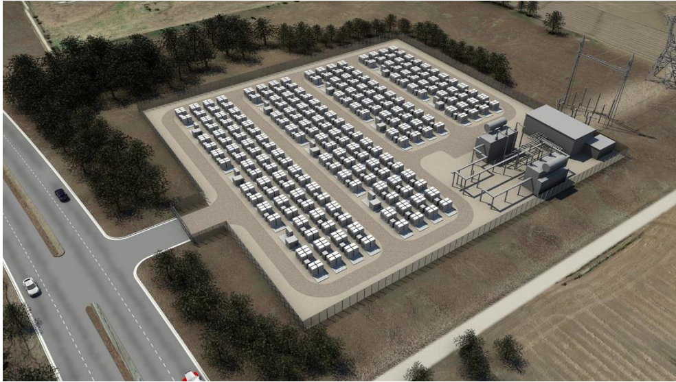
Tesla Grid Storage Facility (Southern California)
