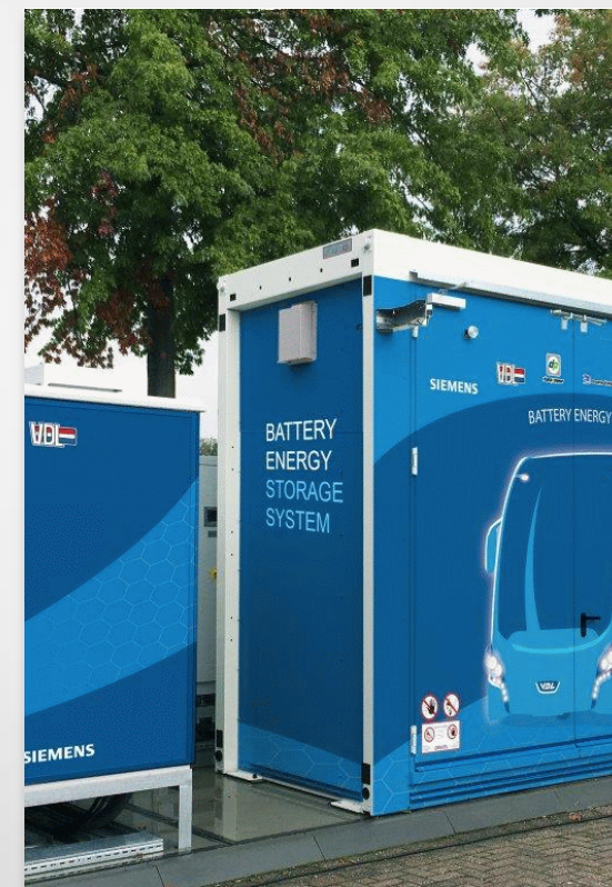
Energy Storage Systems (kW)
