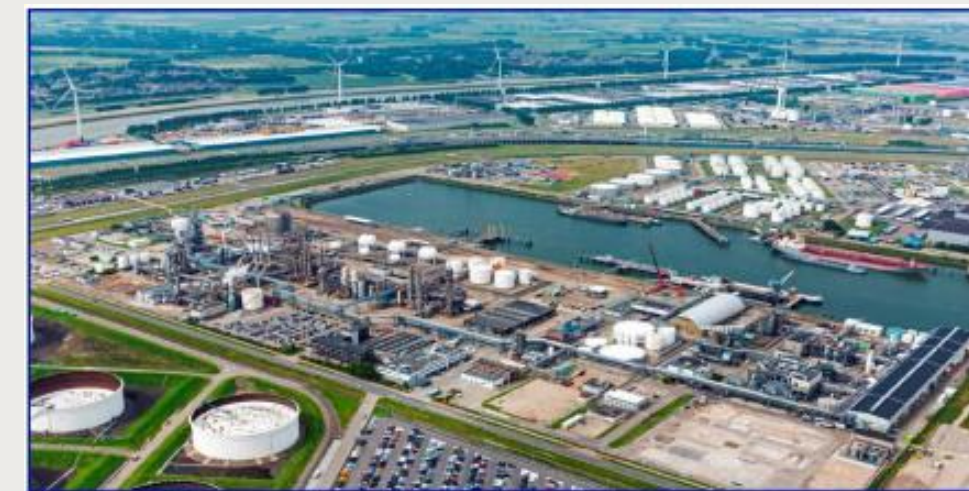
Air Products, Rotterdam (by product H2 from Chlor-alkali process)
