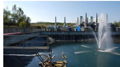
Remo-stort Houthalen From waste via plasma gasification
