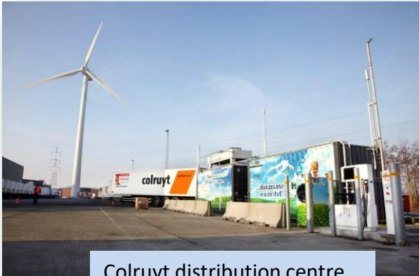
Colruyt distribution centre From wind-solar
