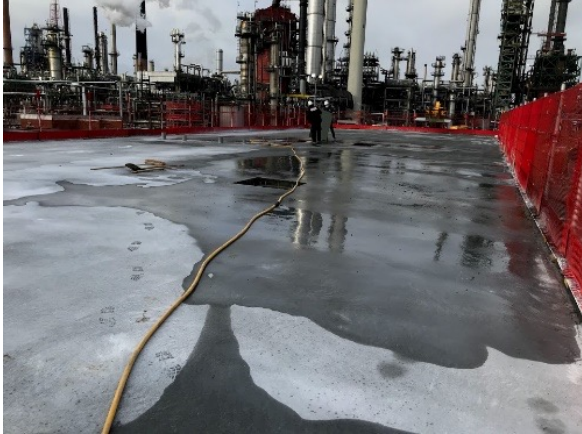
Total New build blast resistant building, offices and work station
