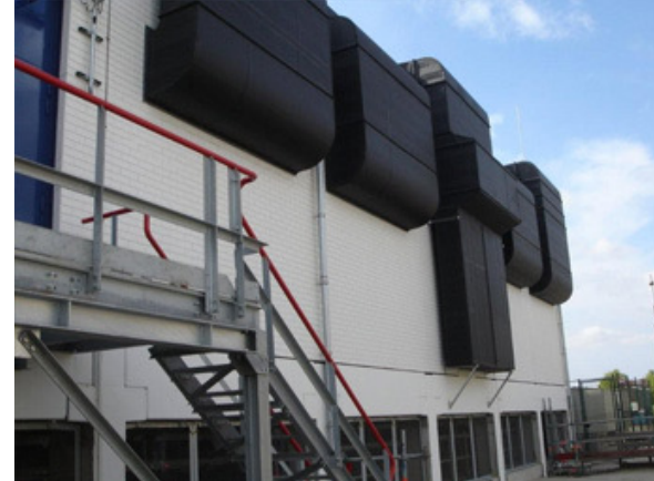
Esso Substation 107 Study, design and construction of a industrial building
