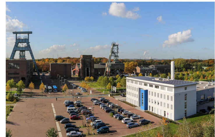
Hydrogen Application Center in Herten
