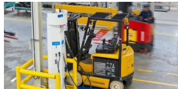
Supply for H 2 forklift trucks
