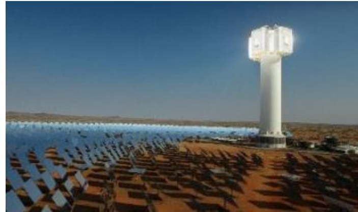
Solar thermal power plant 24/7 thanks to molten salt
