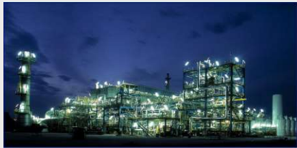
Air Liquide, Port Jerome (SMR +CCS)
