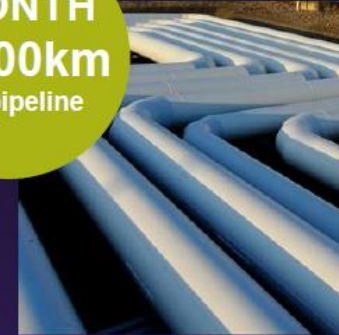
1.4m dia pipe @100bar
