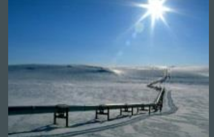
Pipeline Leak Detection System
